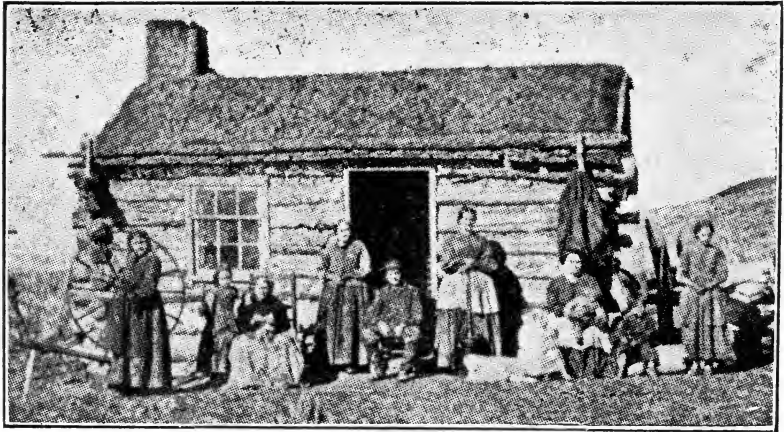
Pioneer cottage. Several families working together.
